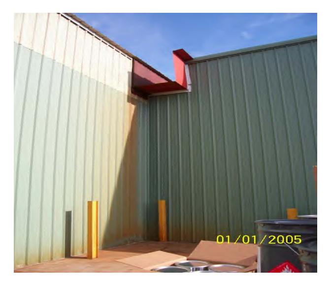
Picture: Internal Gutter 5ft deep.
